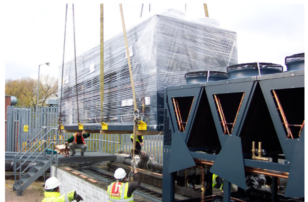
After: A new Turbomiser chiller is lowered into position onsite
