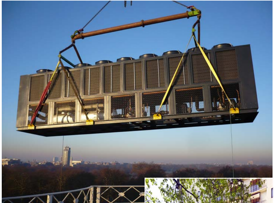
The chiller being craned onto the roof of the Dorchester (above). The prestigious London Hotel (right) now has a combined chiller capacity of 3MW
