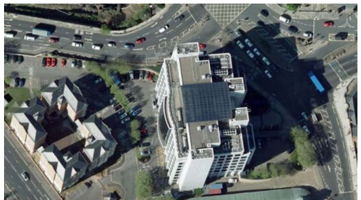
Skandia's landmark building in Southampton is served by two rooftop-mounted Turbomiser chillers
